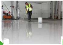
13. After the material has been placed on the prepared substrate, KÖSTER LF-VL can be evenly distributed using a suitable smoothing tool. The material is self-leveling.
