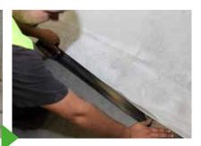
6. Joints and the edges of the work area are taped off to achieve straight edges and to keep the area clean.
