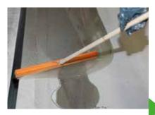
7. KÖSTER CT 121 is used as a primer. Substrates with high vapor drive must be sealed with KÖSTER VAP 2000.
