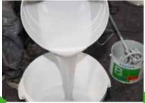
11.To avoid defects due to insufficient mixing, re-pot the material and mix again. The KÖSTER Resin Stirrer achieves even results as a mixer attachment.
