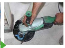
3. Details such as corners and edges have to be prepared by mechanical grinding.
