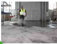
8. Broadcast dried silica sand into the wet primer (only when primed with KÖSTER CT 121) to increase the bond strength of the subsequent layer.
