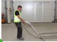
5. To enhance bonding performance all dust and loose particles are removed by vacuum cleaning.
