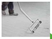
4. When shot blasting is performed with steel abrasive, the surface is cleaned with a magnetic broom. The collected shot can be re-used.
