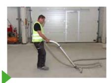
9. After curing, surplus material is removed by vacuum cleaning.
