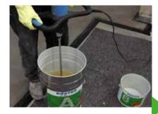
10. The components are mixed for a minimum of 3 minutes with a mechanical stirring device until a homogenous consistency is reached. Follow the mixing procedures given in the Technical Guideline.
