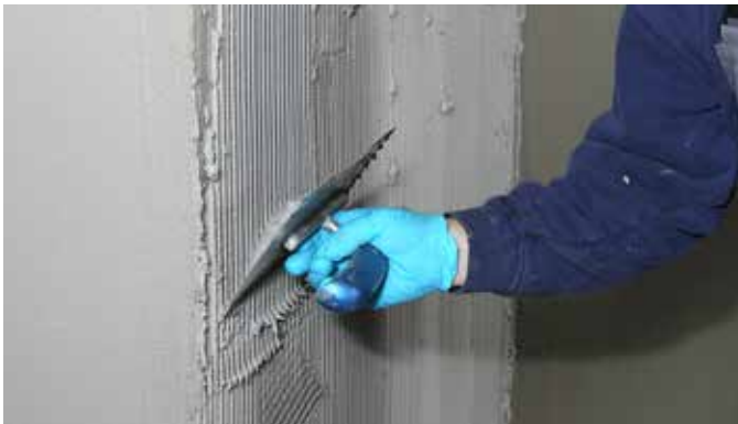
Internal basement waterproofing
