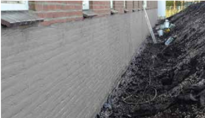
External basement waterproofing
